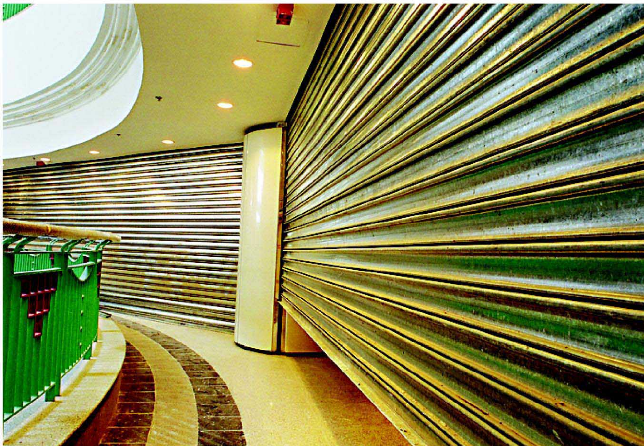
Fire rated shutter in a shopping arcade
